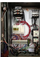
Front opening control panel eliminates the need for 48" side clearance as required by NEC® standards.
