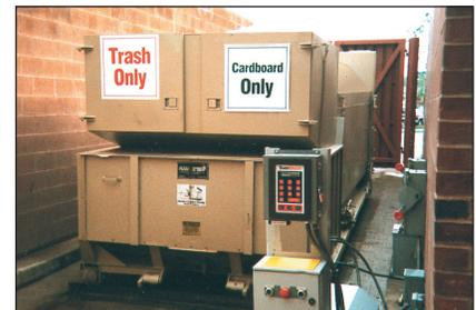
Also available with an advanced system for measuring and reporting container usage and fullness. Users can input an I.D. number to access the compactor.
